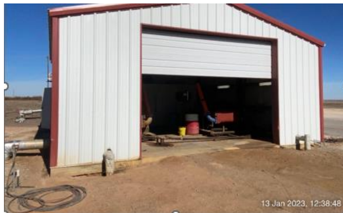
Permanent Wind barrier
