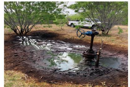
This abandoned well was found in a retention pond for a new housing development in the Houston area. RRC's well plugging program eliminated the threat the well presented to the Lake Houston watershed and area homes. The total cost for plugging this well was \$110,000.
