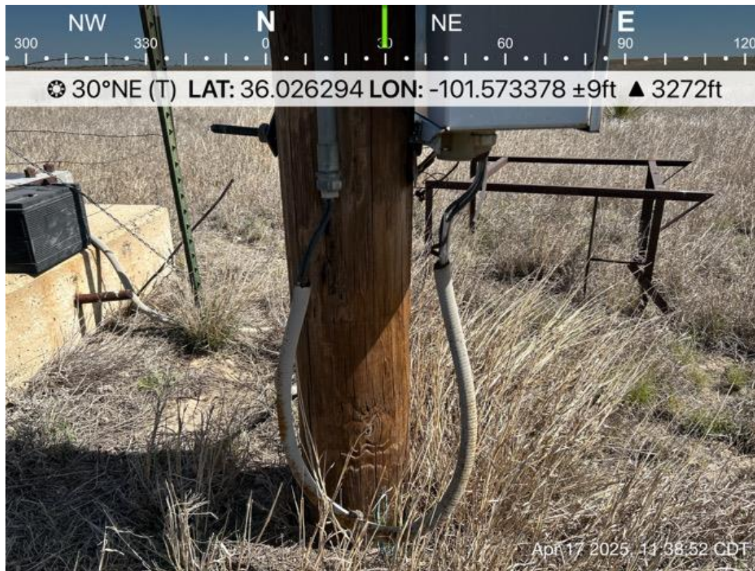
Wires are Exposed Conduit Disconnected
