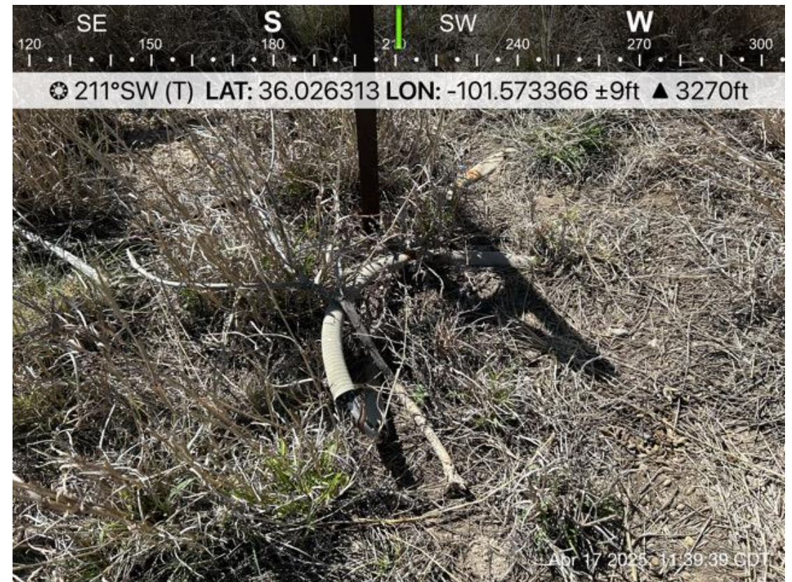
Conduit is Split Exposing Wires
