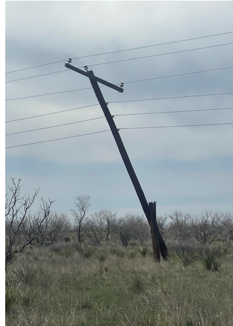
Condition of the Pole = Hazardous Condition for Lines
