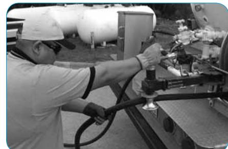
Inspecting Delivery Hose Assembly After Each Delivery
